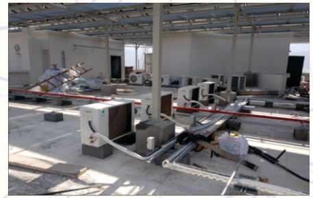
Installation of 30 Nos Split A/c for IT & Electrical rooms
