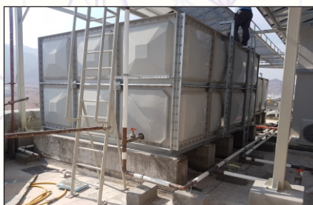
GRP TANK Installation of GRP Tank on the roof top. Total capacity of 40,000 Ltrs
