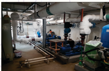
Chiller Pump Room - Installation of two sets of Chilled Water Pump along with Chilled Water Piping with Primary and Secondary Pumps
