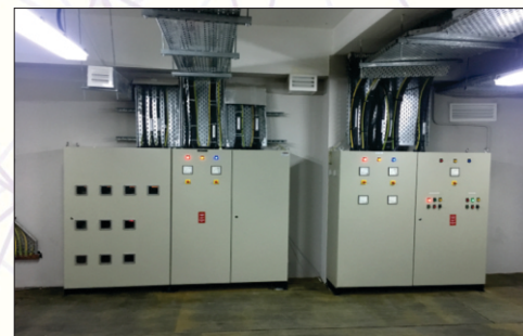
Oasis Mall LV Room - Laying of Cables
