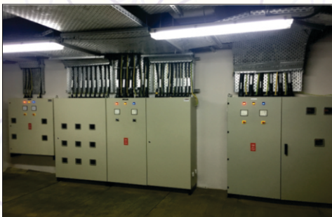
Oasis Mall LV Room - Laying of Cables
