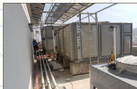
GRP TANK Installation of GRP Tank on the roof top. Total capacity of 40,000 Ltrs
