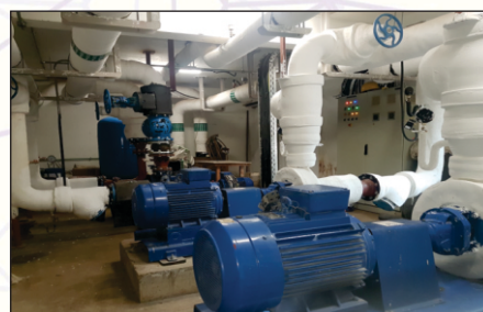
Chiller Pump Room - Installation of two sets of Chilled Water Pump along with Chilled Water Piping with Primary and Secondary Pumps
