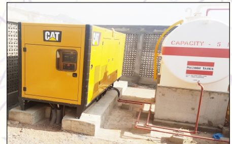
Installation of 550 KVA Generator & Diesel Tank Capacity 5000 Ltrs
